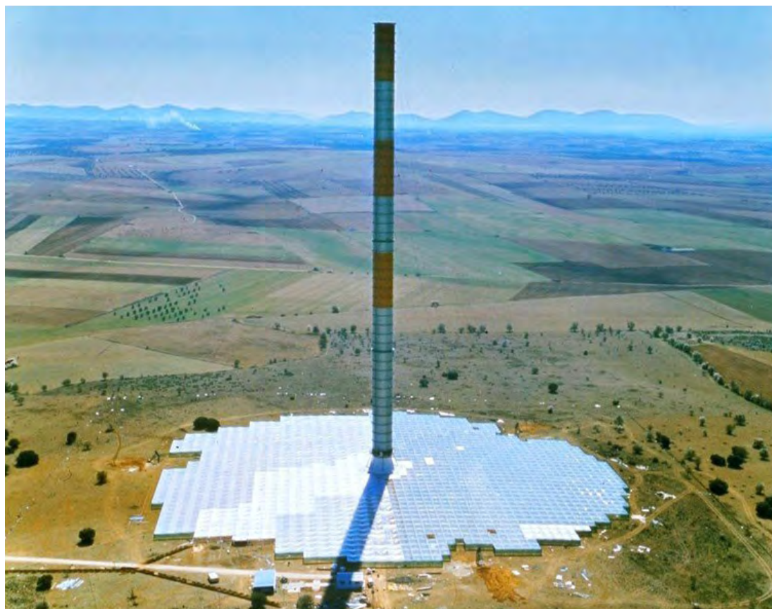
Pilot plant in Manzanares
