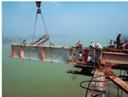
Second Hooghly Bridge in Kalkutta, 1970 - 1992
