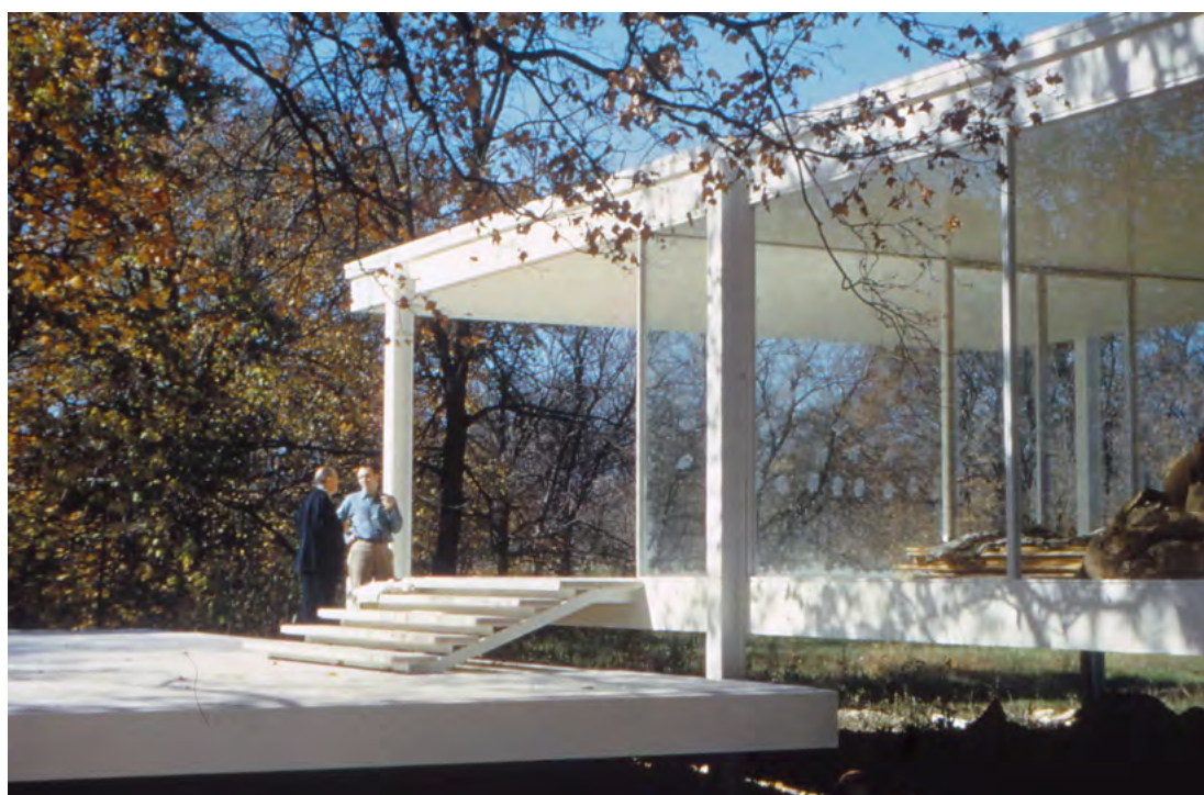
Mies van der Rohe (left) visits the Farnsworth House construction site with project supervisor Myron Goldsmith. (Photograph taken by architect Y.C. Wong)
